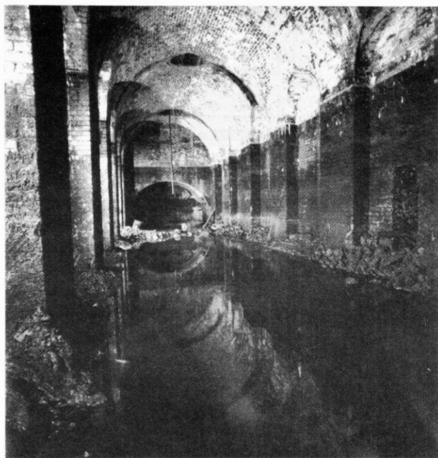
Plate 3 Rope-tensioning vault with well at end for counterpoint (BWCP)
